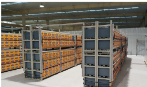
Photovoltaic, EV Charging and Battery Energy Storage System
