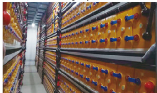
IDC Backup and Battery Energy Storage System
